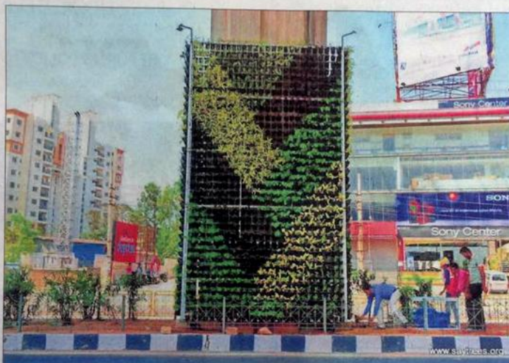
A vertical garden on a pier of the flyover at Pragathi Nagar, Electronics City.
